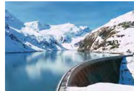
Pumped Storage Power Plant Kaprun
