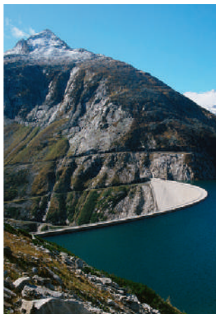
VERBUND's power plant at Malta
