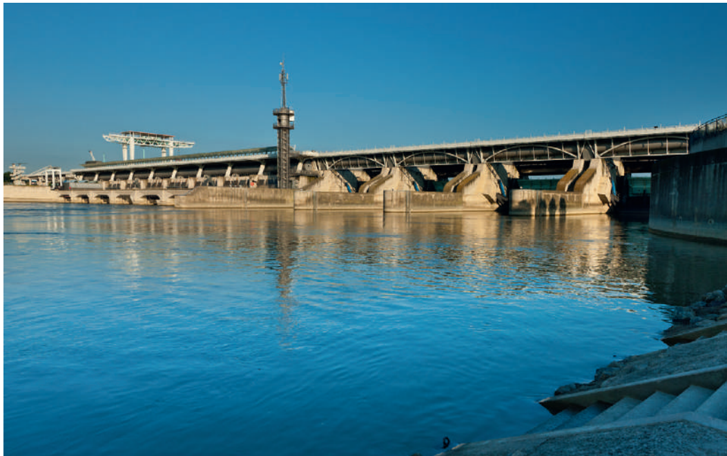
VERBUND's run-of-the-river power plant of Freudenau
