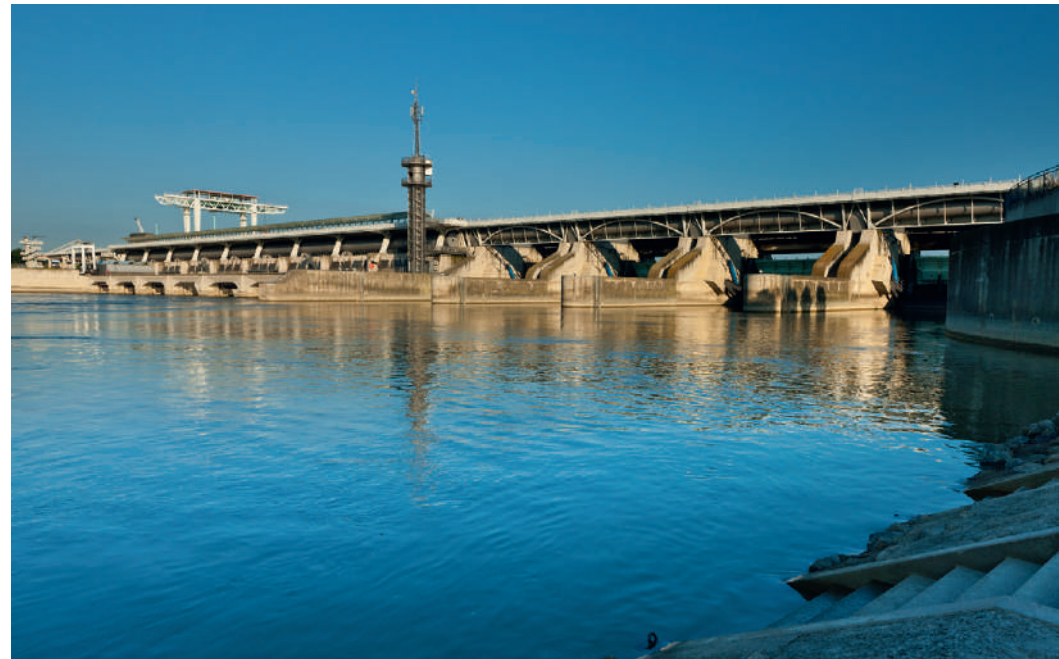
VERBUND’s run-of-the-river power plant of Freudenau
