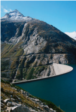
VERBUND's power plant at Malta
